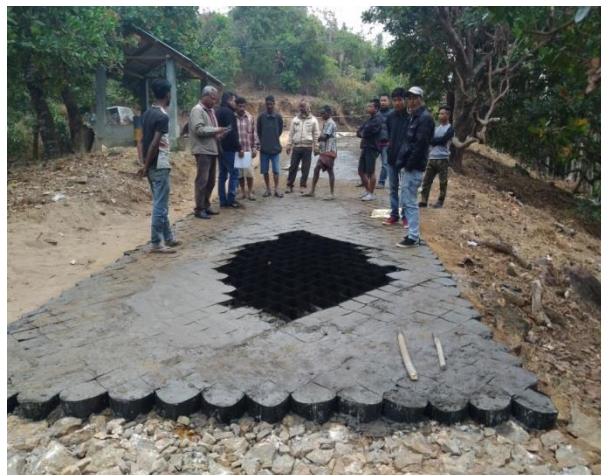
Plastic Cell Technology Road at Ellengre, South Garo Hills, constructed through convergence with MGNREGA
