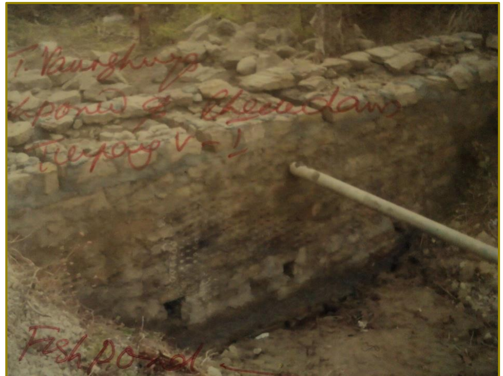
Construction of Check Dam
