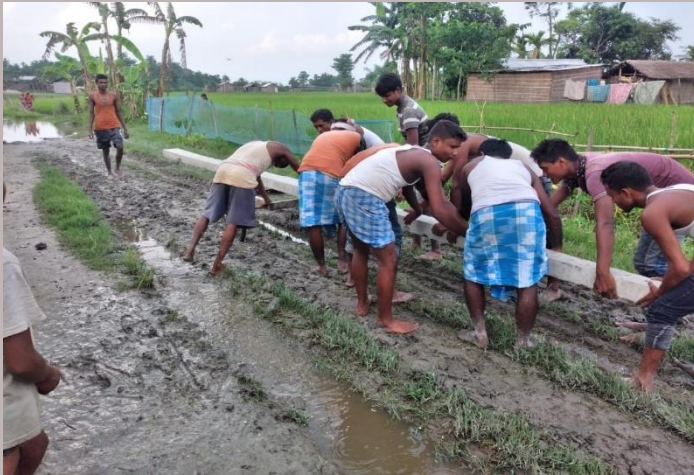
Electricity Poles movement for installation
