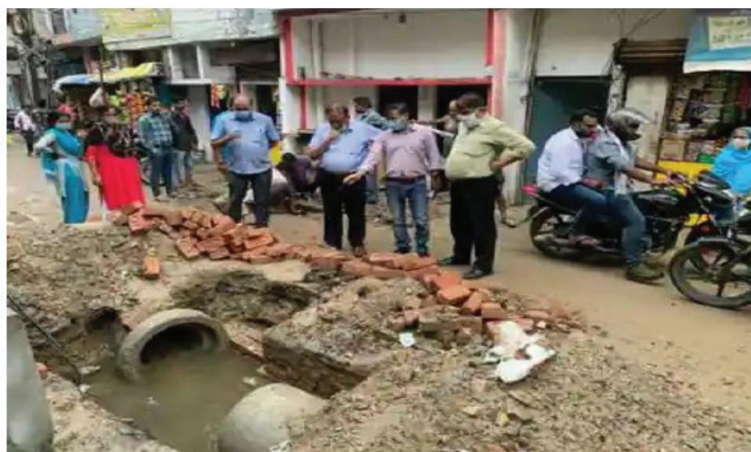
Fig. 1: Damaged sewer line resulting in contamination of drinking water supply
