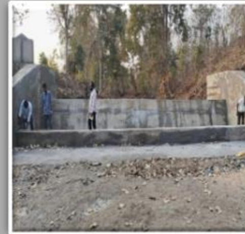
Construction of Check Dam at Khampur for Water Management
