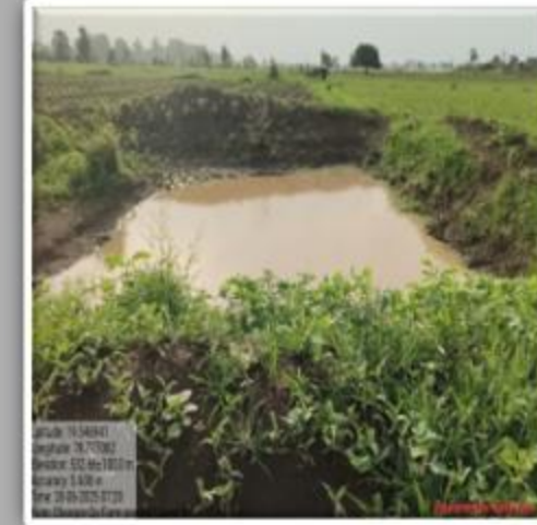
Percolation Tank at Chorgaon GP – Built under JSJB
