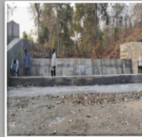
Construction of Check Dam at Sungapur for Water Management
