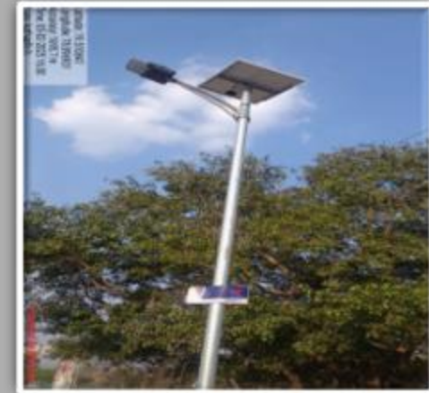
Installation of Community Street Lights with support of BAIF
