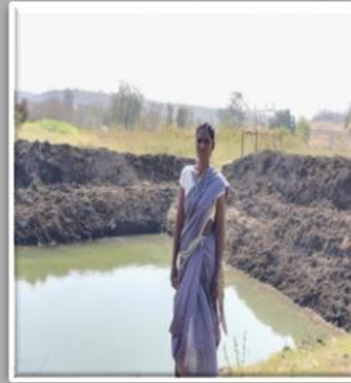
Construction of Farm Ponds in fields
