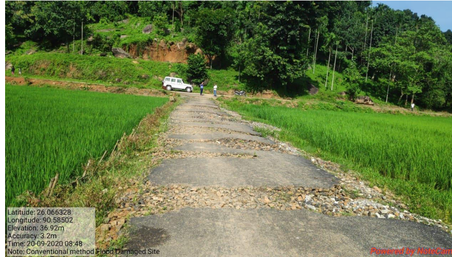
Less Damage to Cell Filled Road
